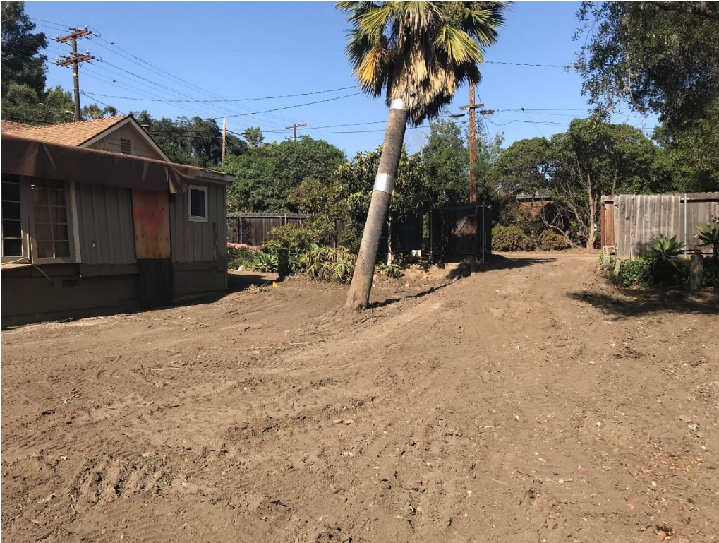
Image 5: 1257 After Debris Removal (view from southwest)
