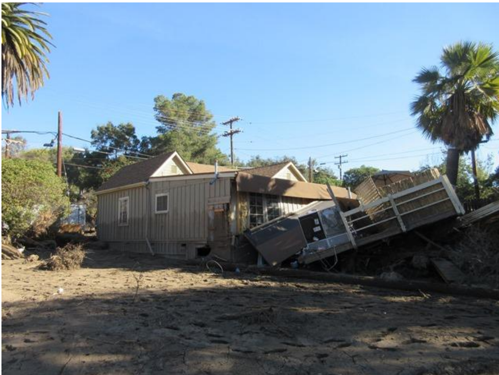
Image 4: 1257 Before Debris Removal (view from southwest)
