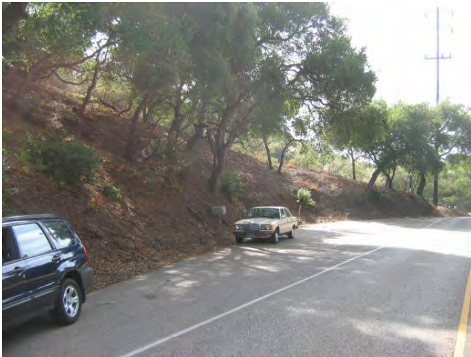
Site D facing west along East Valley Road. Note steep slopes and coast live oak trees.
