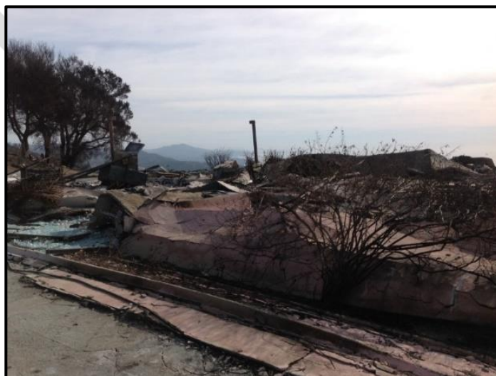
Hot Springs Lane - PDU destroyed
