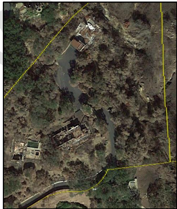
East Mountain Drive - post-Thomas Fire (Source: Google Earth)
