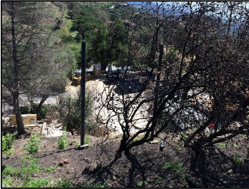
East Mountain Drive – PDU and ADU were destroyed
