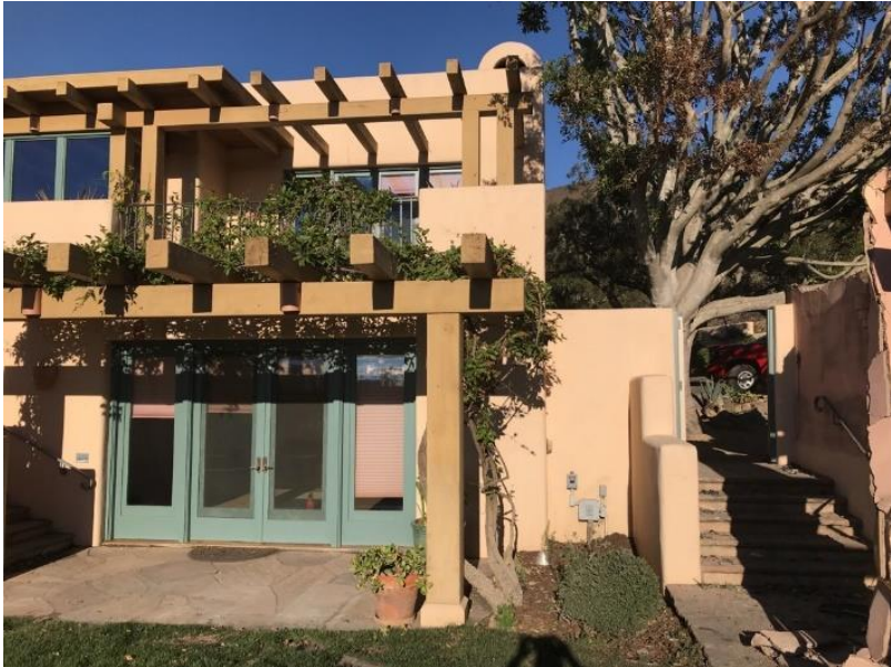
Hot Springs Lane - ADU was destroyed but the PDU survived
