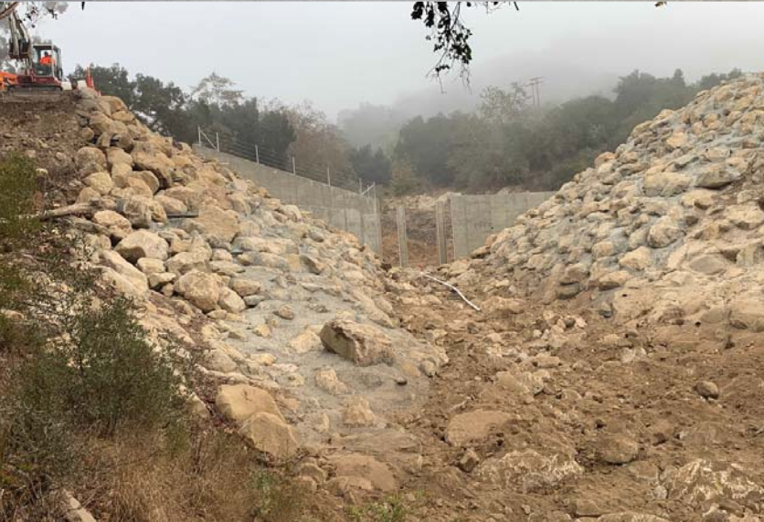
ROMERO DEBRIS BASIN CONSTRUCTION
