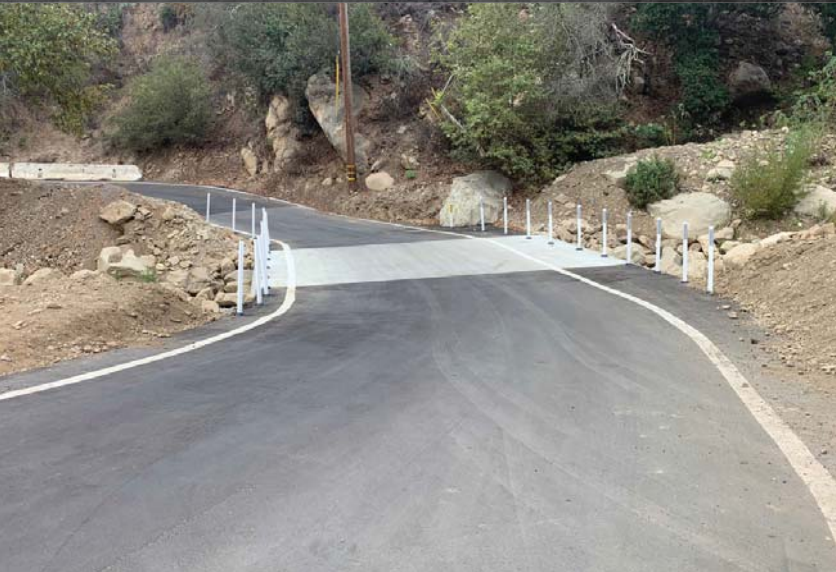
ROMERO CREEK CROSSING UPGRADE
